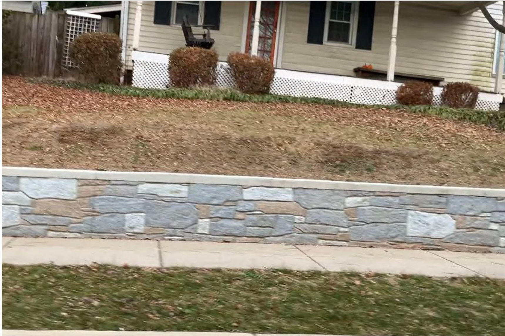
Hyattstown along Frederick Rd Constructed Retaining Wall
