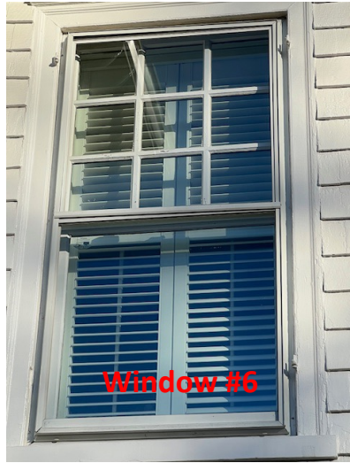
Side View (Facing East from Driveway – 2 nd Floor)
