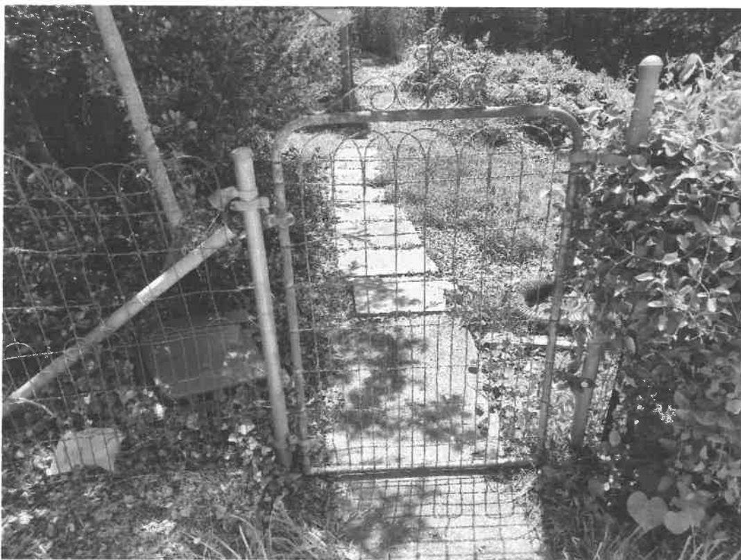
Typical walkway gate existing, Baltimore St
