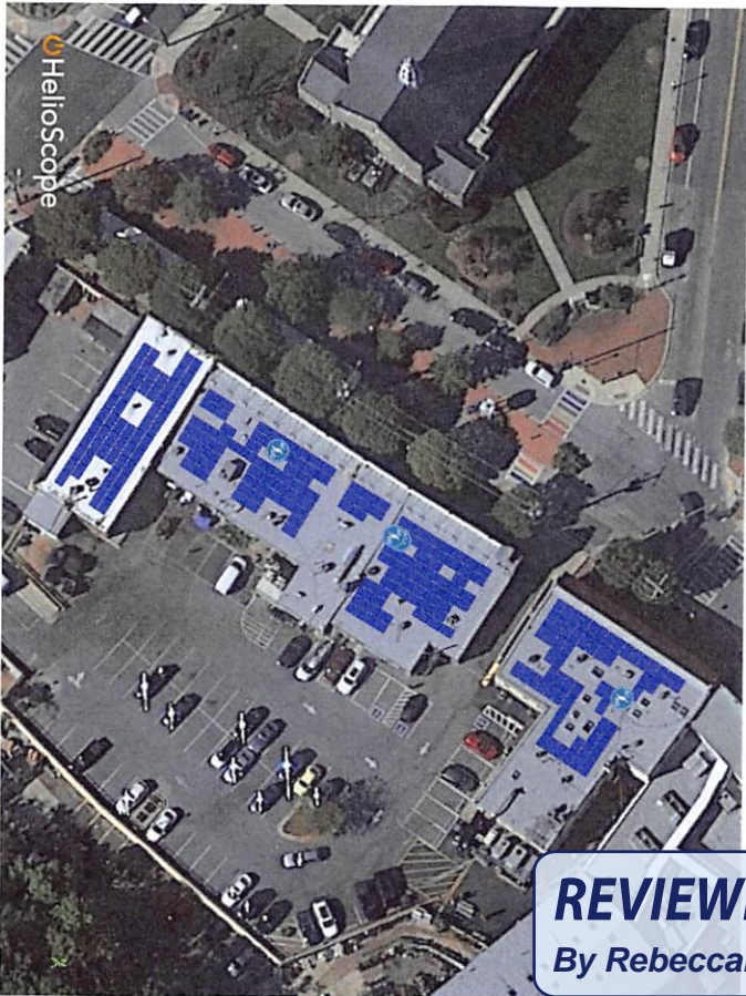
Preliminary design and system capacity subject to revision during detailed engineering study
