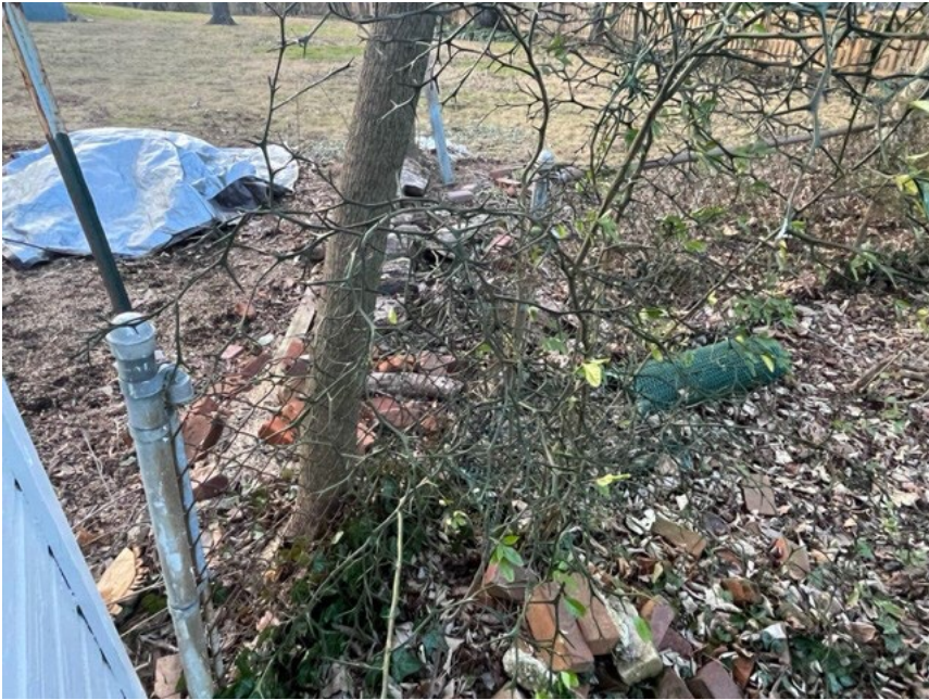
Back yard west side existing fence to be replaced, photo 2
