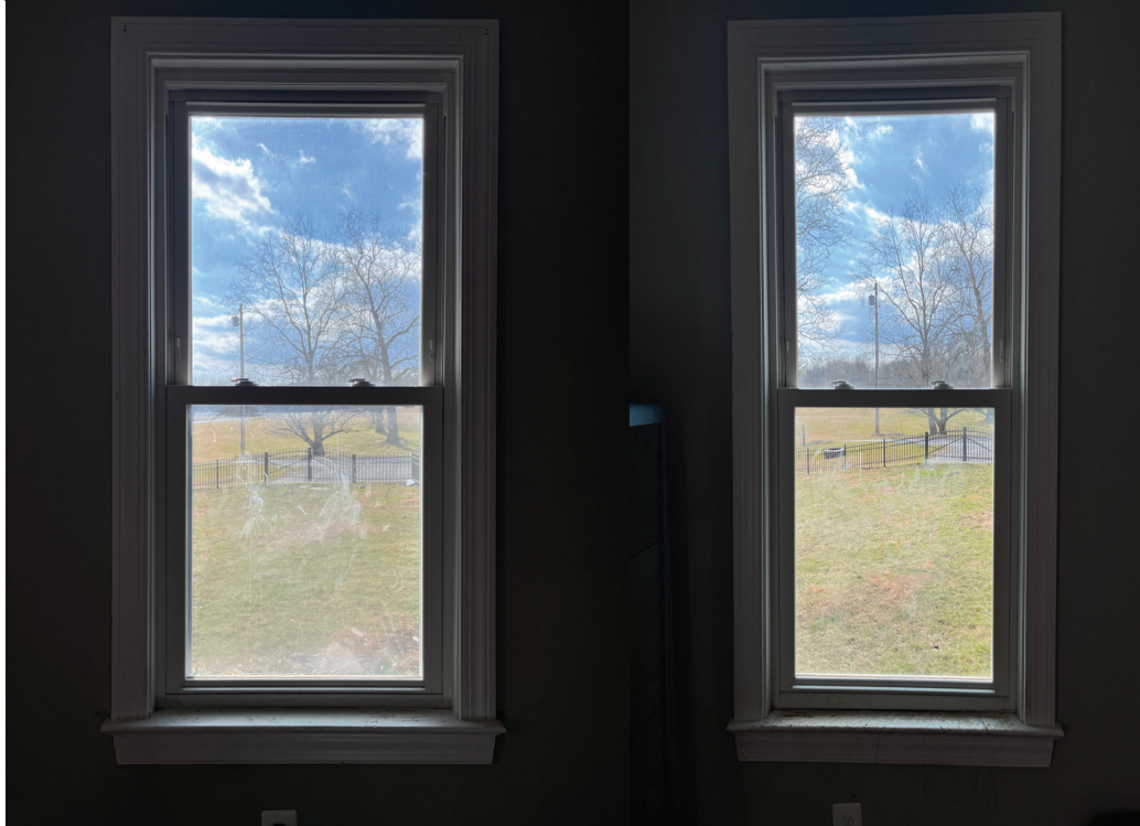
Interior and exterior photos of office windows to be replaced
