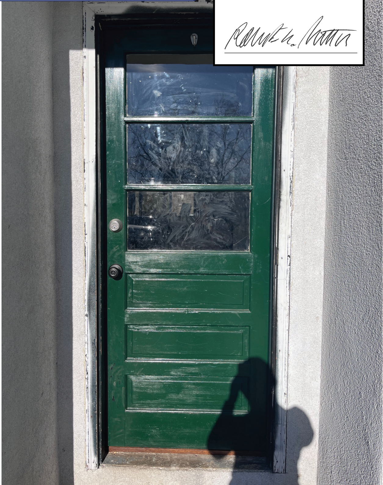
Exterior front door with wooden frame painted white (storm door had been damaged in windstorm and removed).
