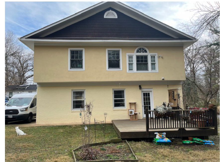
4. SOUTH ELEVATION - REAR OF EXISTING STRUCTURE
