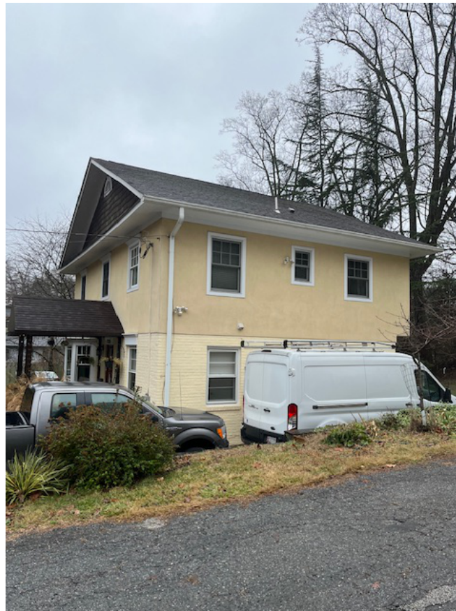
2. EAST ELEVATION - SIDE OF EXISTING STRUCTURE
