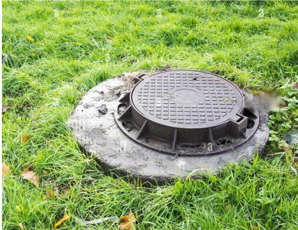
Photo 3: Example manhole cover.
