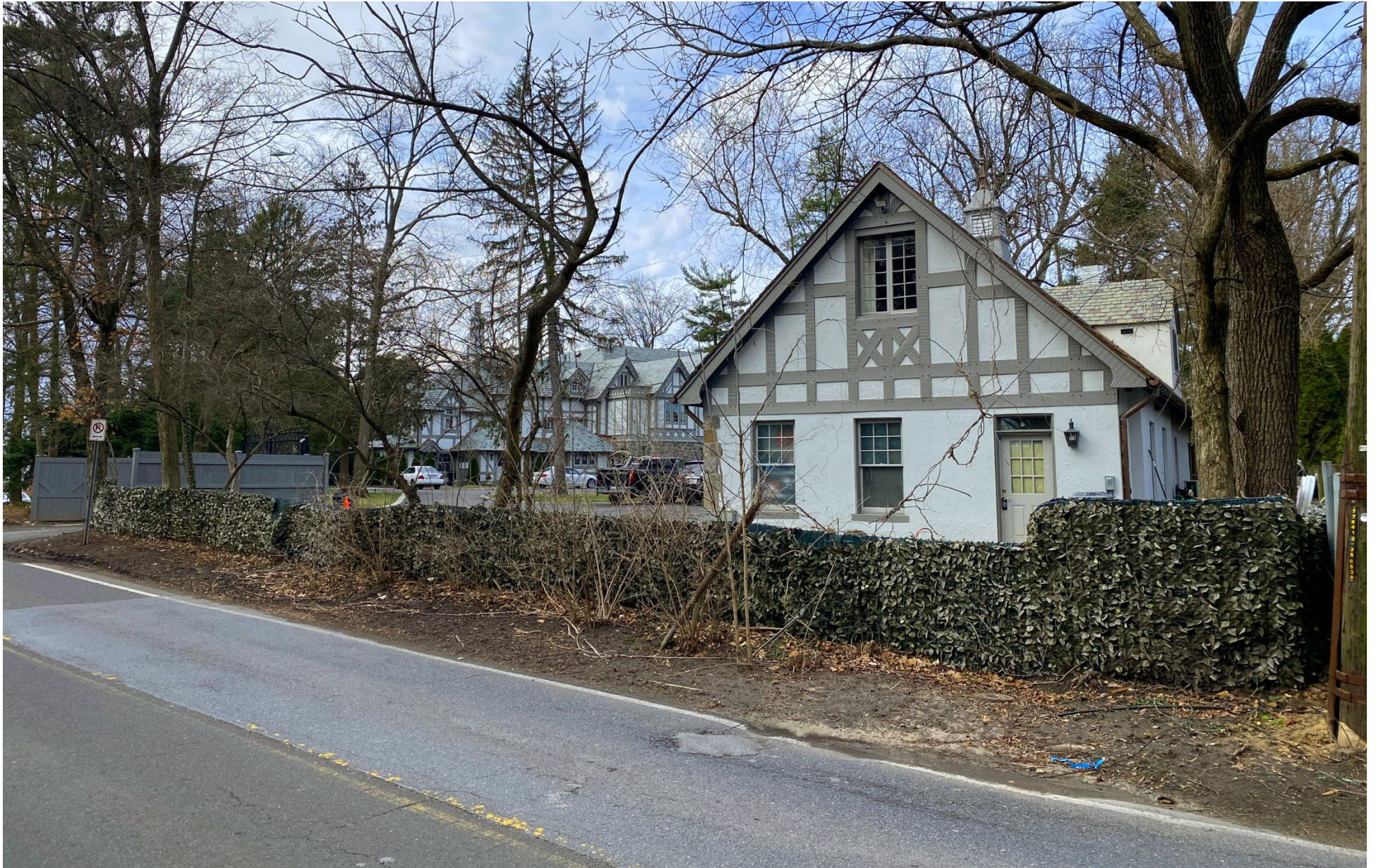
Current fencing and view of main house from Brookville Road.
