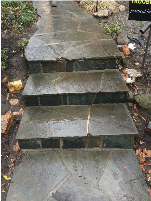
EXISTING STEPS AT SIDEWALK & WALKWAY
