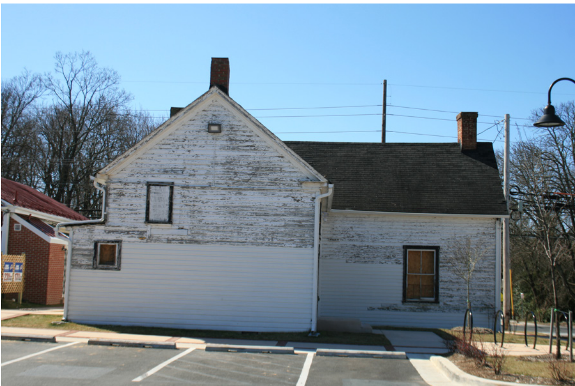
Photo 03 Rear Facade (East Elevation) Photo by Ward Bucher | March 01, 2020
