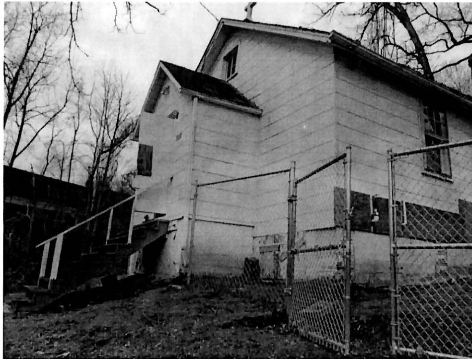
Photo No. 5: View of the front entrance as seen from the northeast corner. Note that the structure is wood-framed and clad with painted asbestos wall tiles and asphalt roof shingles.
