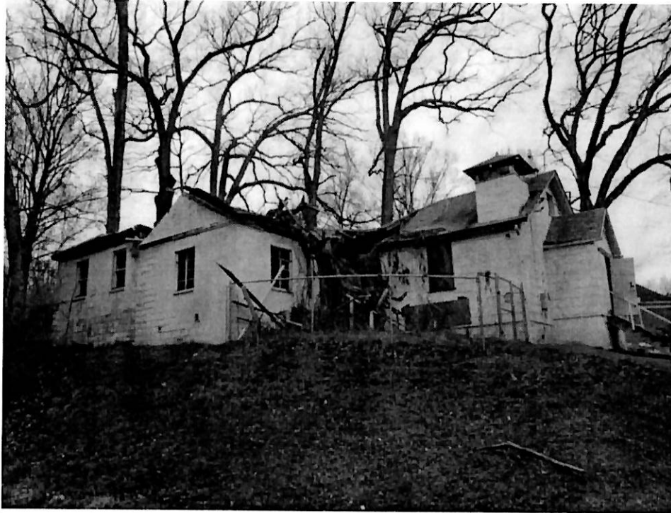
Photo No. 9: General view of the structure's southeast corner as seen from the level of the streambed to the south. Note that the roof of the structure's southwest has been completely collapsed; however, the front portion of the structure (including front entranceway and bell tower) remain intact.
