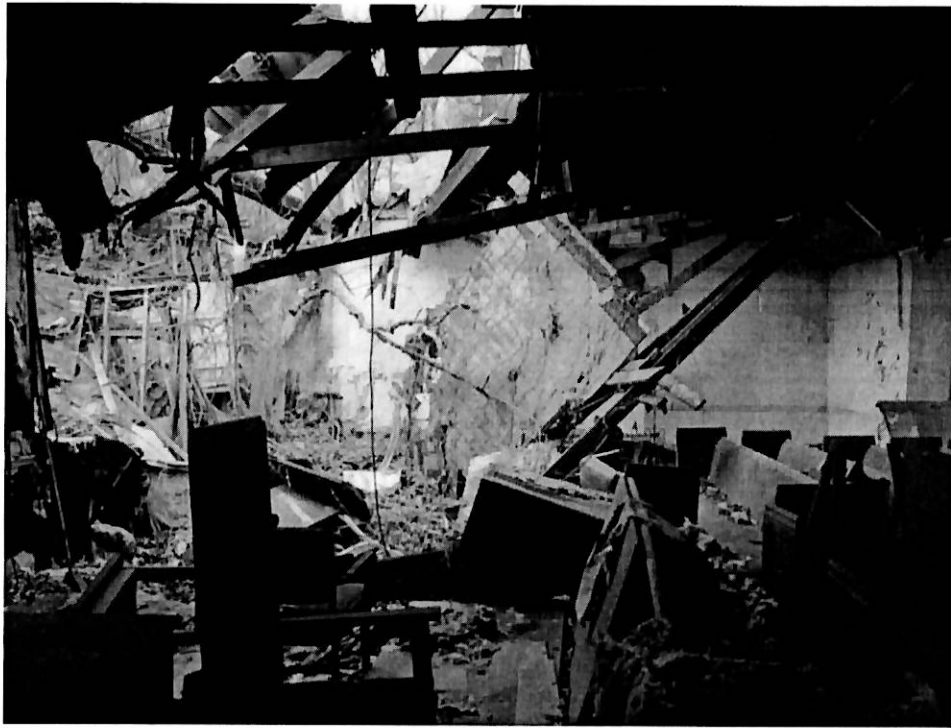
Photo No. 11: Interior view of the structure (looking west from the front entranceway), exhibiting the collapsed roof of the southwest corner.
