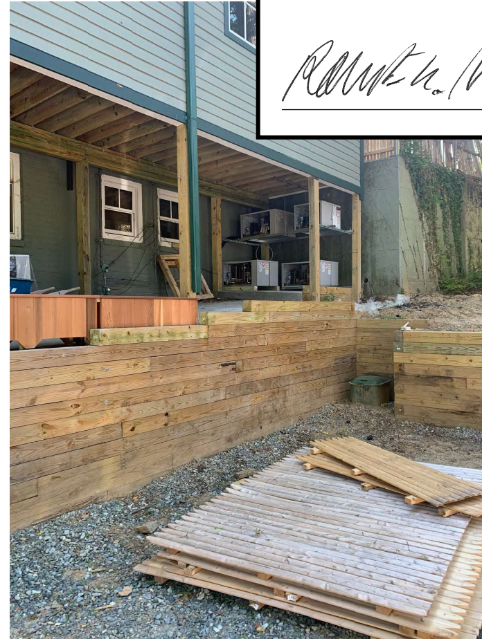
Existing conditions under addition
