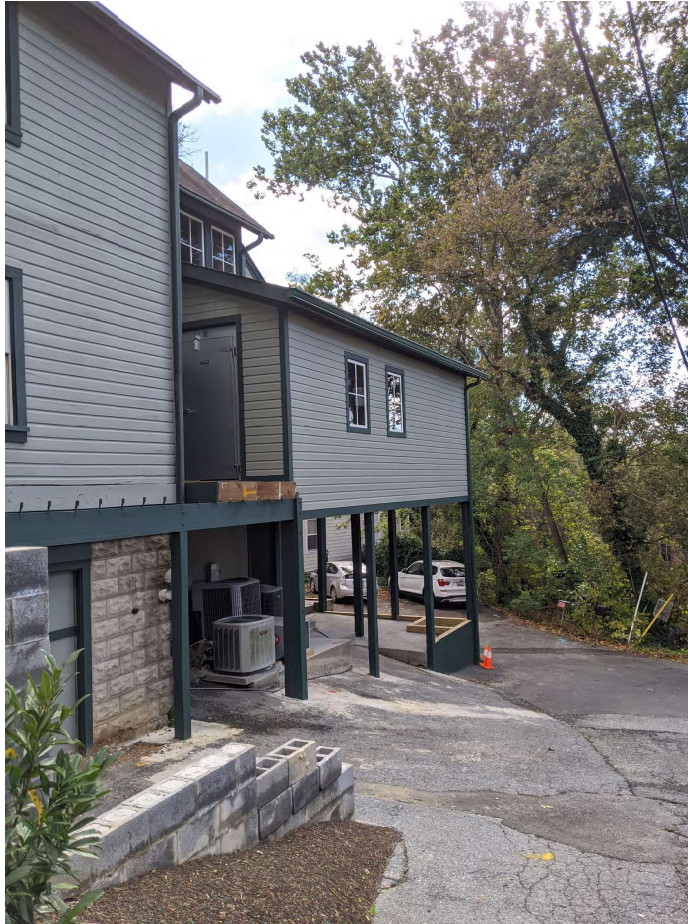
View down Windward from Macarthur
