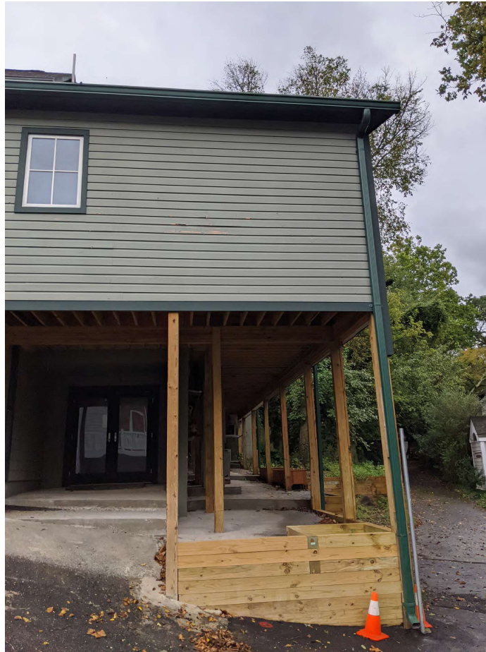
Existing conditions under addition
