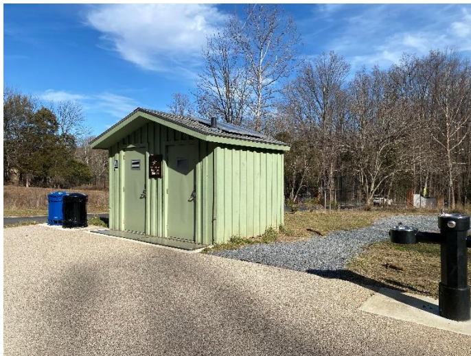
Existing Composting Toilet Bathroom Structure
