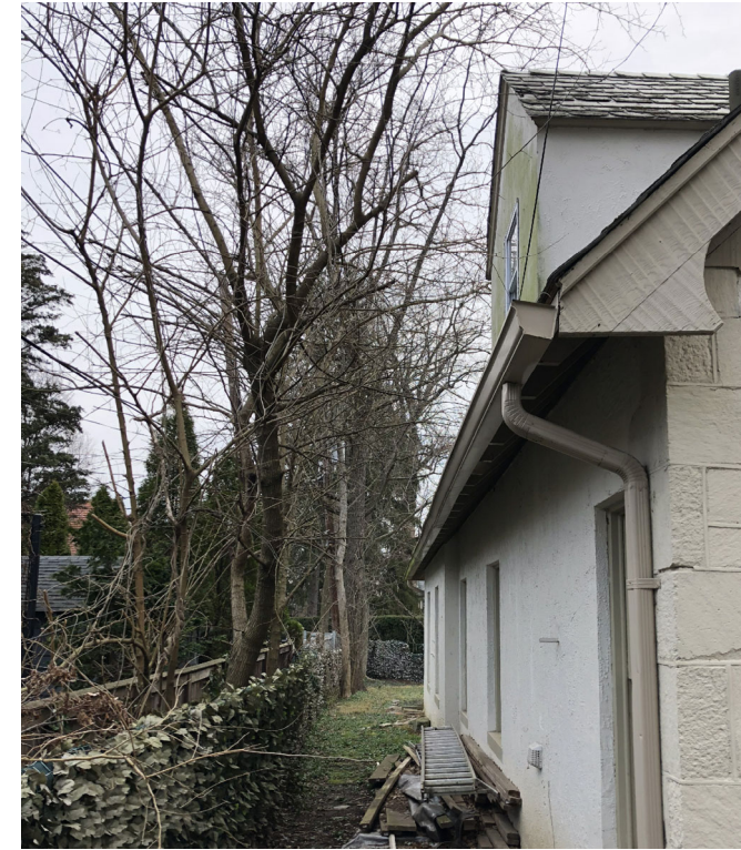
B2 - EXISTING GARAGE DORMER
