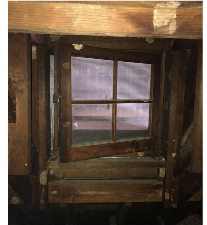
B3 - EXISTING GARAGE WINDOW BEHIND LOUVERS
