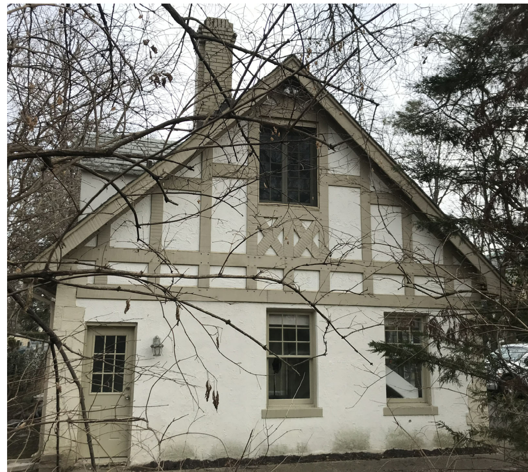
B5 - EXISTING WEST FACADE
