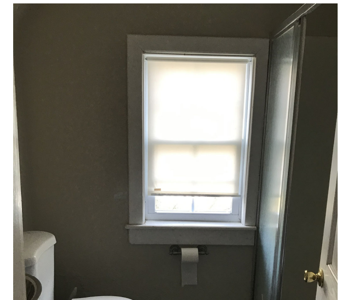
B6 - EXISTING GARAGE VINYL WINDOW
