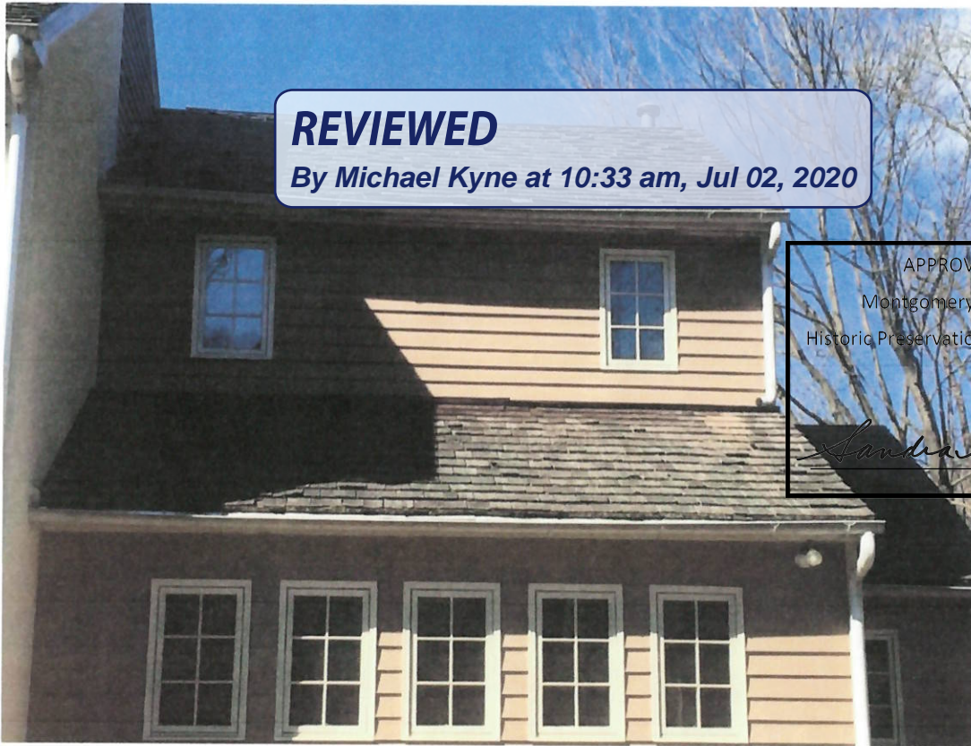
Damaged Shingles 1
