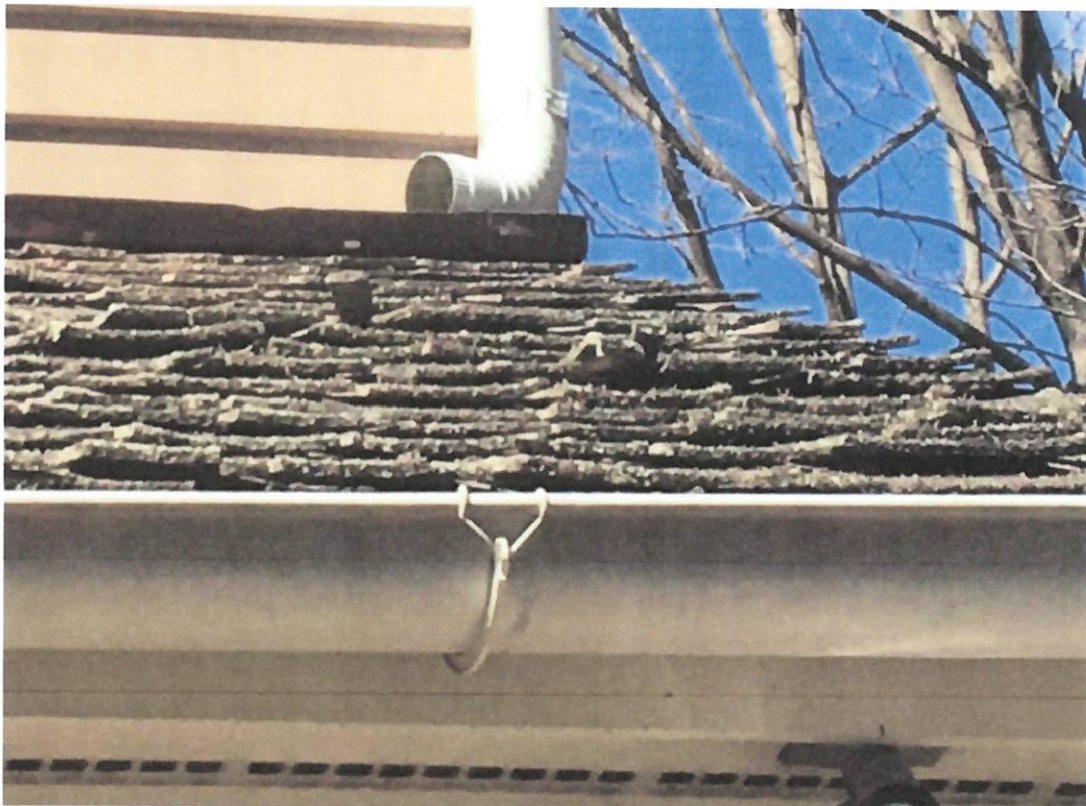
Damaged Shingles 2
