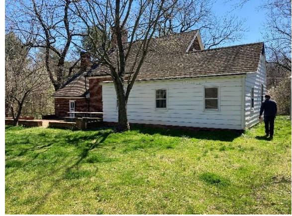
View from rear yard toward rear elevation of the house, from approximate location of proposed shed.
