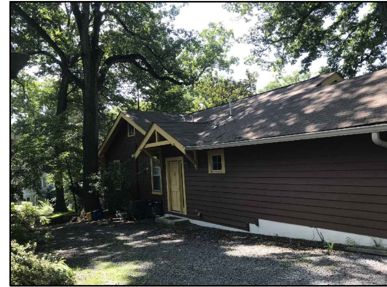
Residence North View (July 2019)
