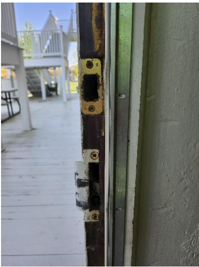
Photo 25-2: 1850s Block Door Jamb, Adjacent Rm 106
