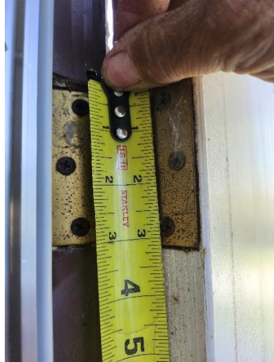
Photo 25-3: 1850s Block Hinge
