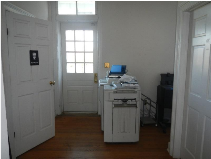
Photo 25-1 1850s Block, Rear Door
