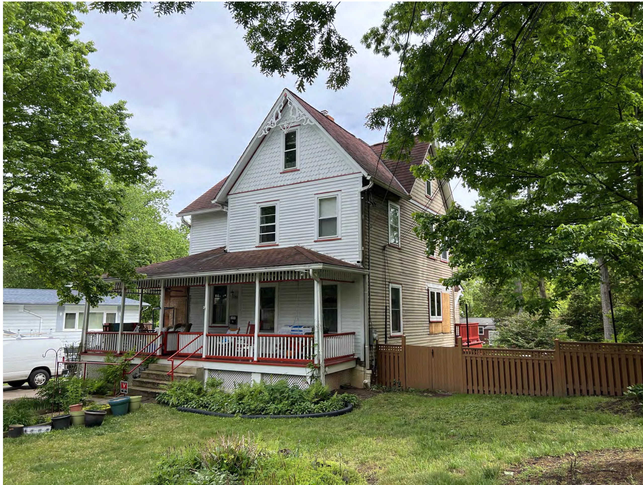
Existing conditions looking at North(Front) and West(Side) Facades
