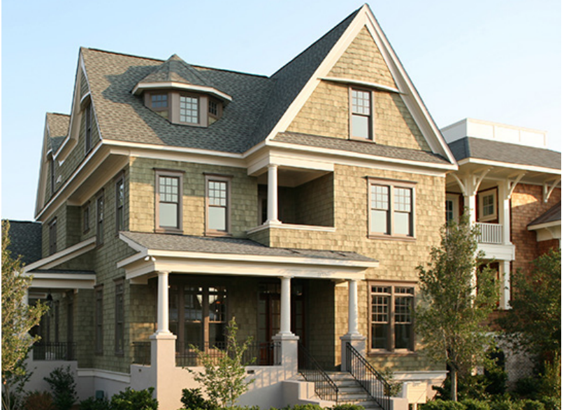
Project: Smith Show Home Location: Charleston, SC Architect: The JD Smith Company Builder: Simonini Builders Product: 7-1/8" Staggered Panels Color: Leward
