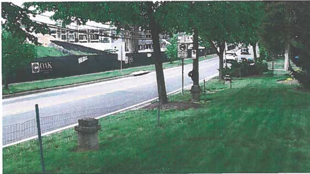
9310 Brookville Road 7-Front, facing Brookville Road Existing wire fence to be replaced
