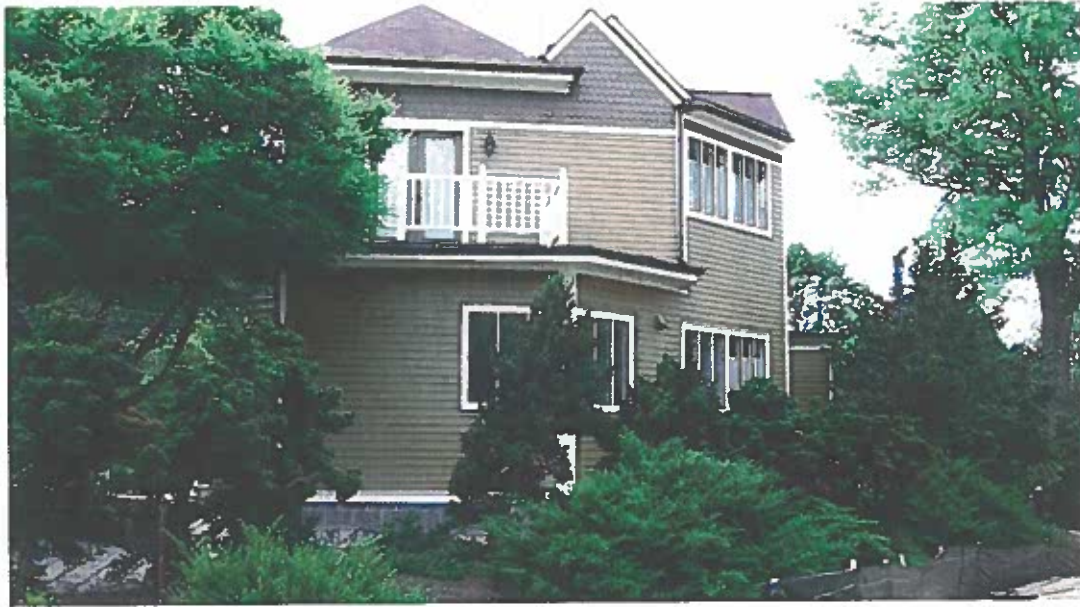
9310 Brookville Road 5-West facade
