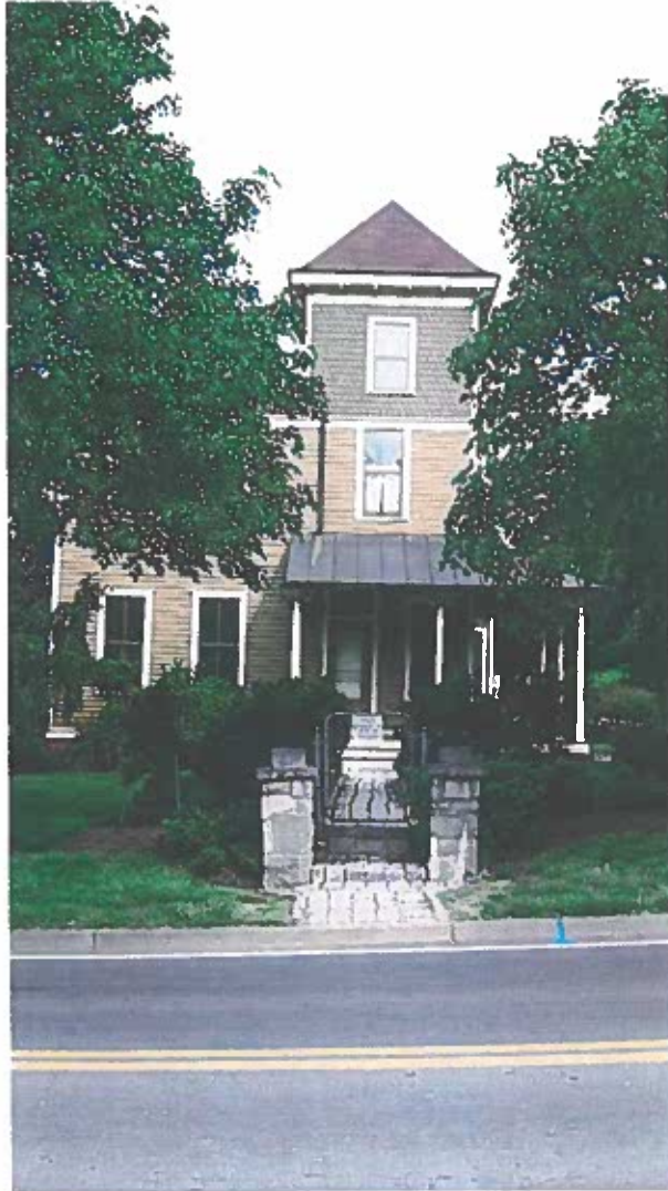
9310 Brookville Road 1-Front facade
