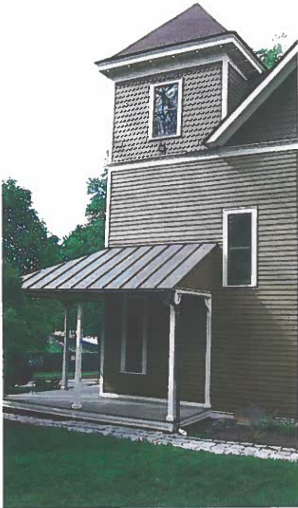
9310 Brookville Road 3-North facade-turret and porch
