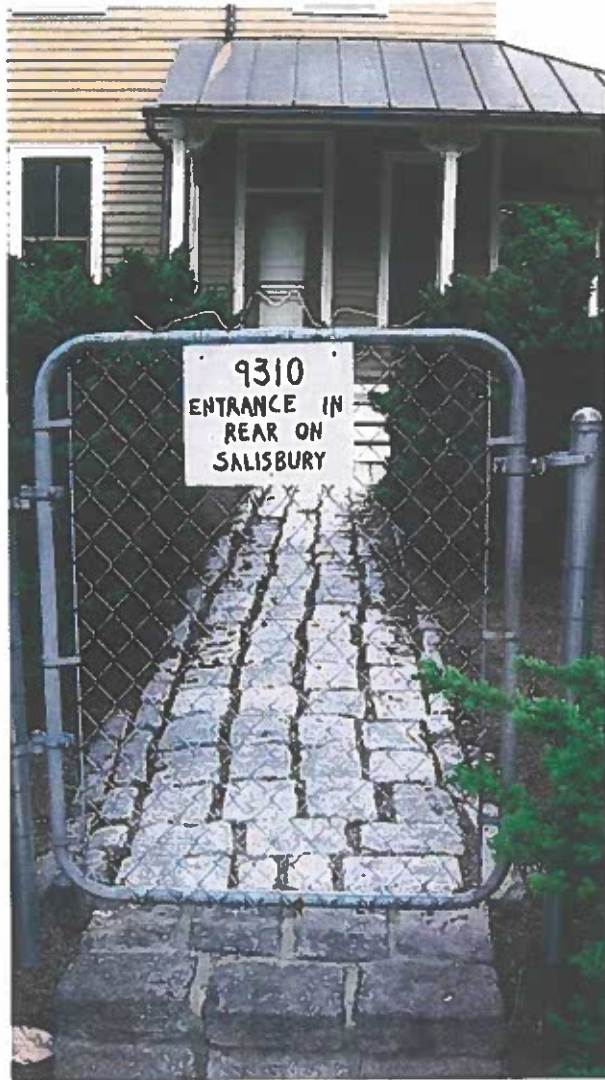
9310 Brookville Road 8-Front-Existing pedestrian gate to be replaced
