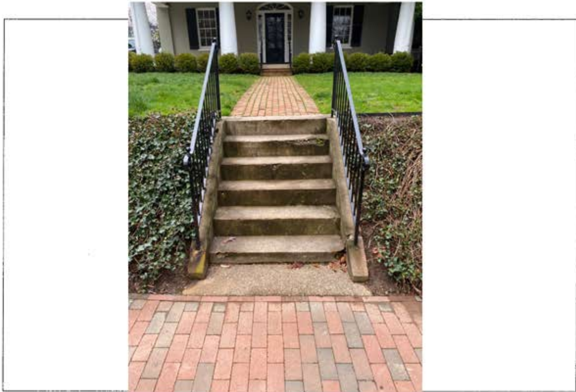
Detail: View of the existing Steps from the street curb
