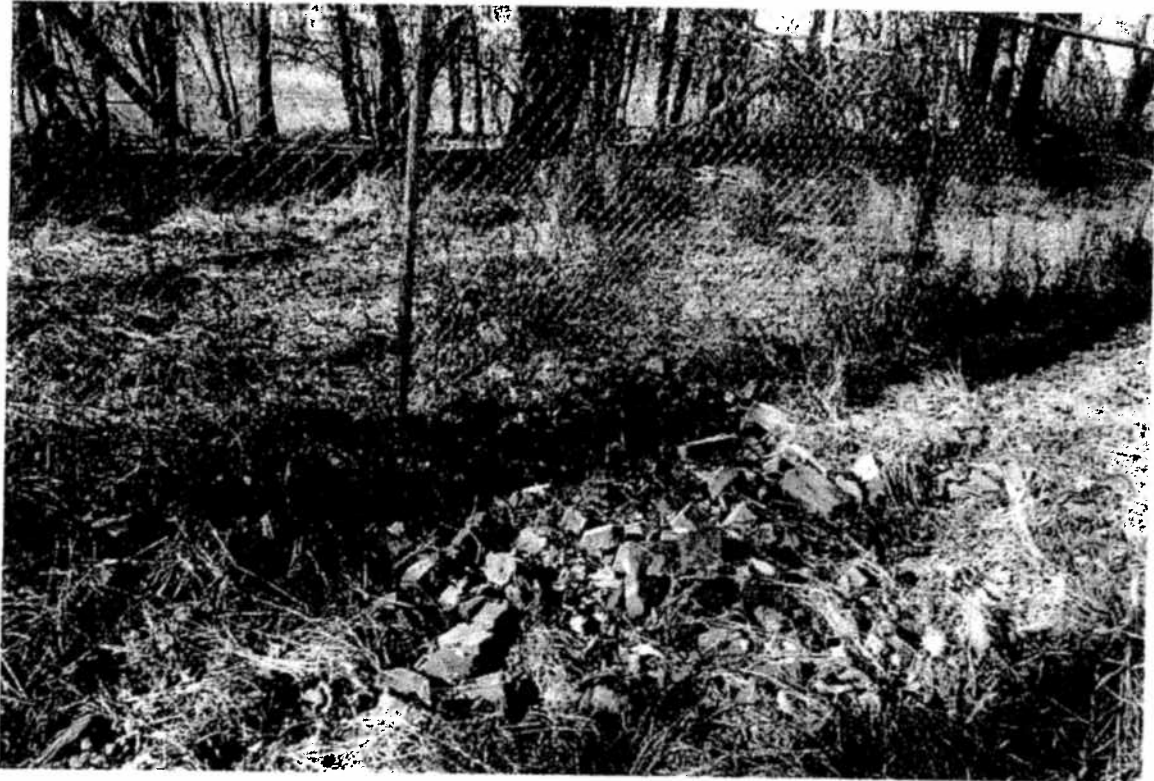
Figure 6. Chimney fall and fire debris, west side of Cashell farmhouse, December 2011.
