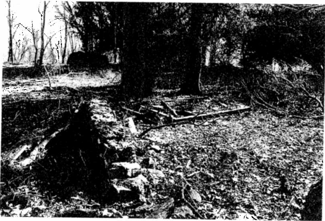
Figure 18. Agricultural outbuilding ruins located east of the farmhouse ruins. December 2011.
