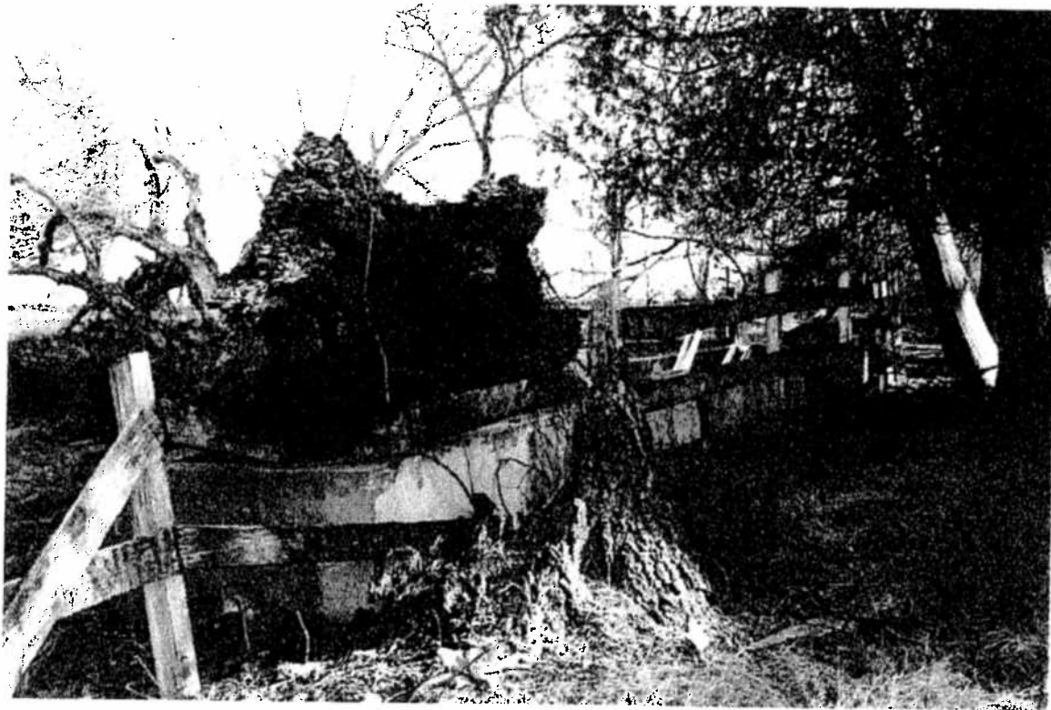
Figure 20. Concrete trough and wood fence north of the stone house. December 2011.
