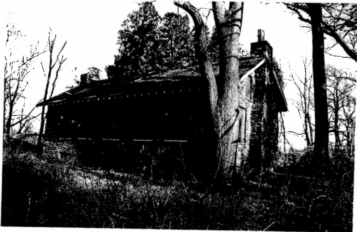
Figure 15. Stone house, December 2011. Rear (west) facade.
