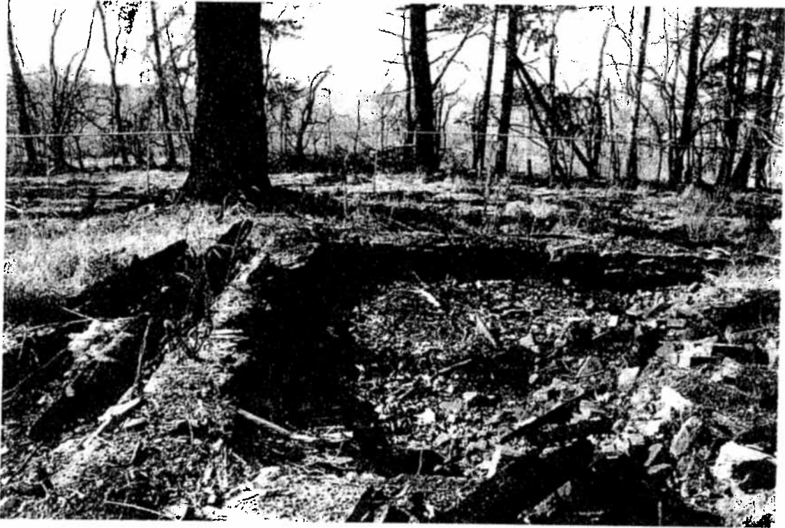
Figure 3. Masonry foundation ruins, December 2011.
