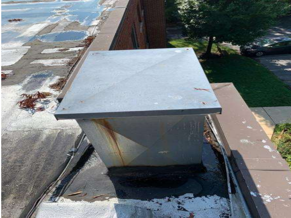
Picture #32 - 1 roof hatch with manual lid
