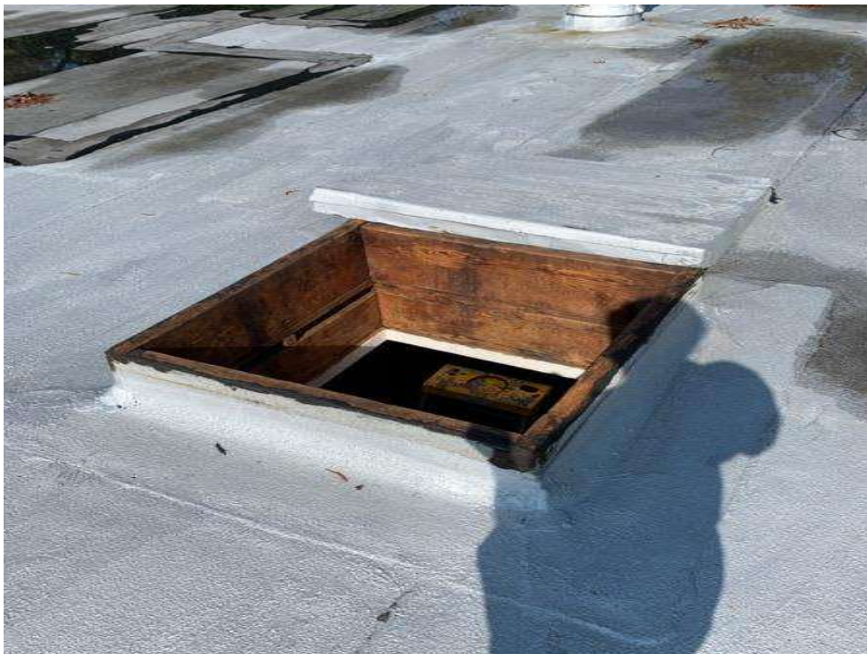
Picture #32 - 1 roof hatch with manual lid
