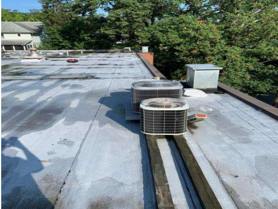
Picture #4 - Significant amount of ponding water
