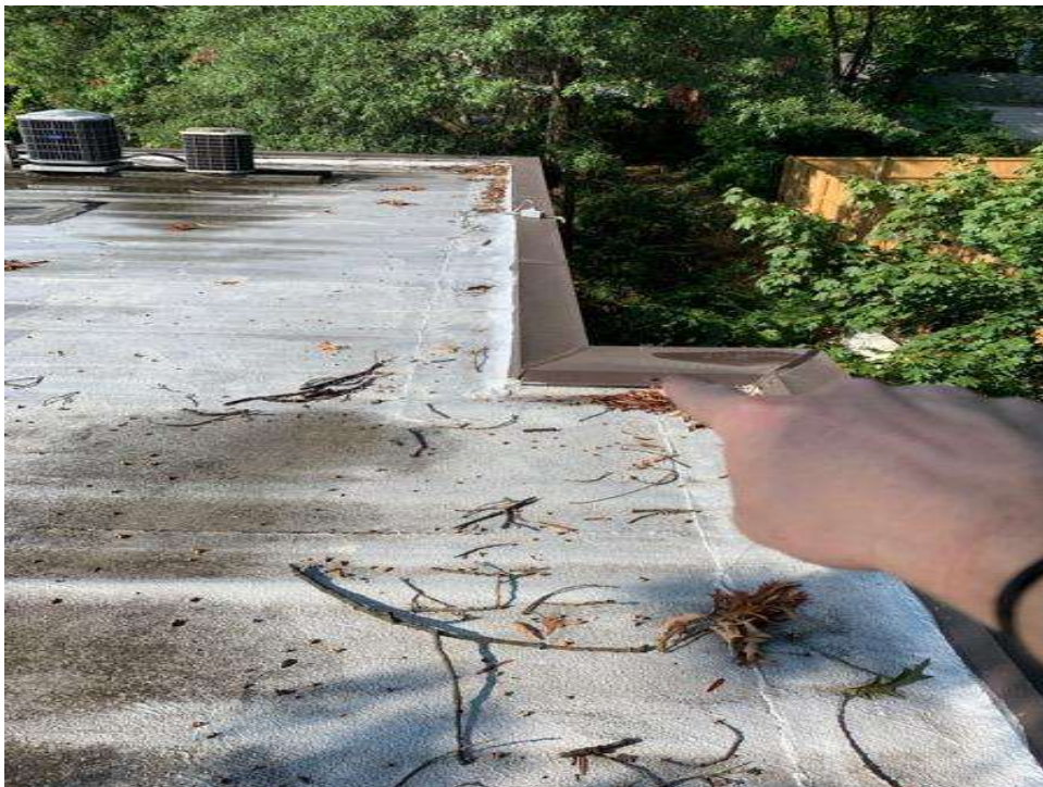
Picture #12 - low parapet heights
