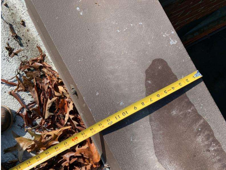
Picture #12 - low parapet heights
