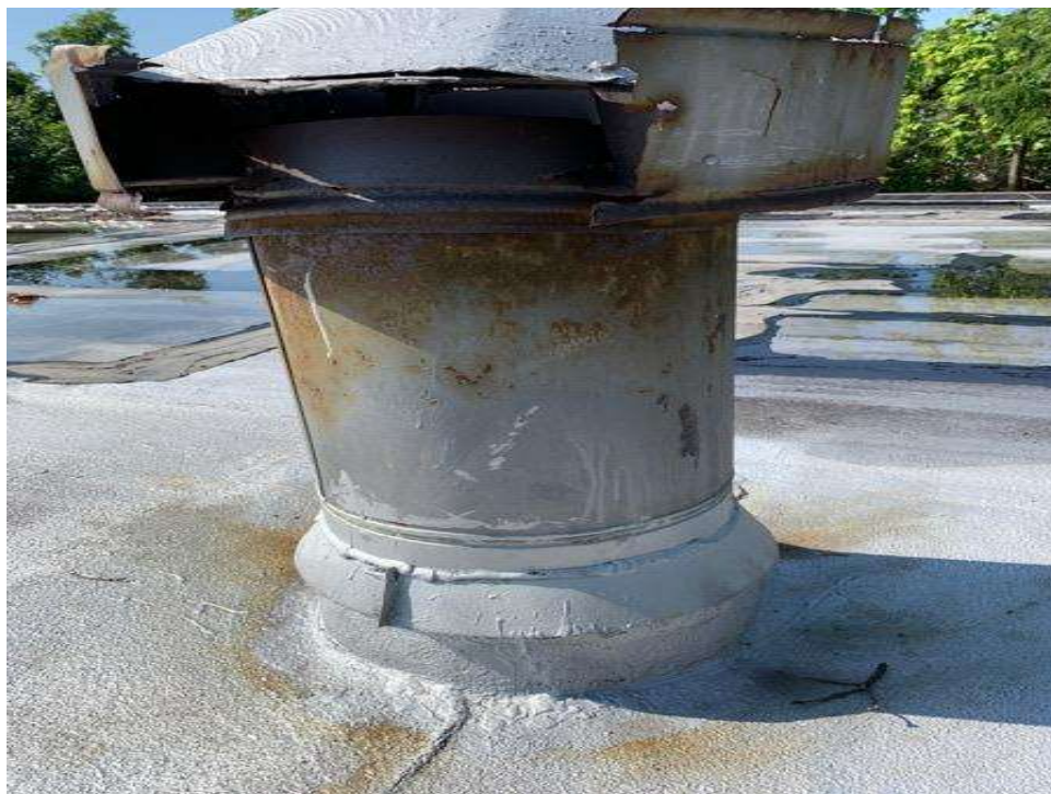
Picture #30 – rusted furnace stack
