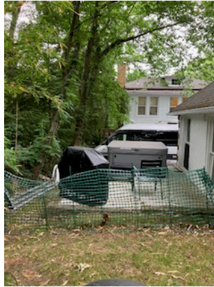
Debra Fuller's New Fence Installation
