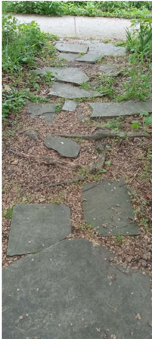
Portion of walkway
