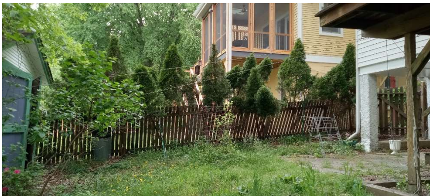
Partially-collapsed wooden portion of fence
