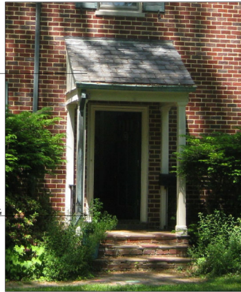
EXISTING FRONT PORCH
