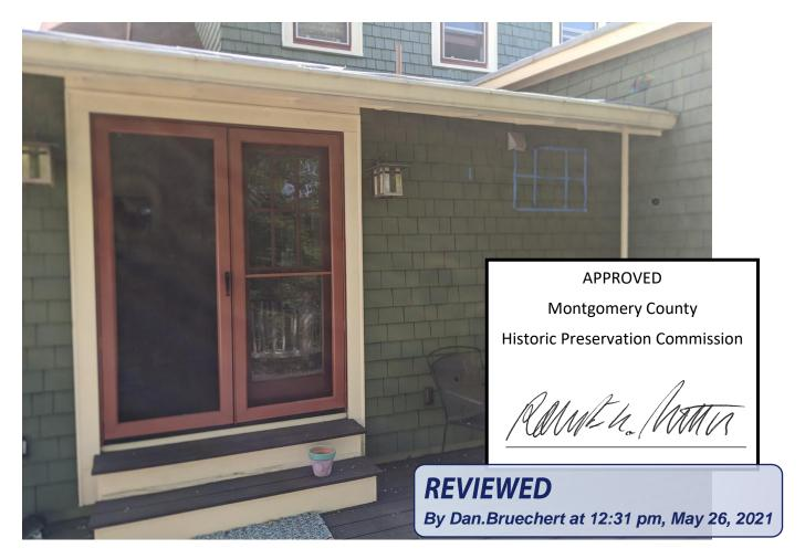
The awning-style window (as shown with blue tape) will have divided light to match the windows in the house. The window will be wood with painted exterior and divided light to match existing windows and doors. Proposed size is 28" wide and 20" high. The window in this addition will not be visible from the street.
