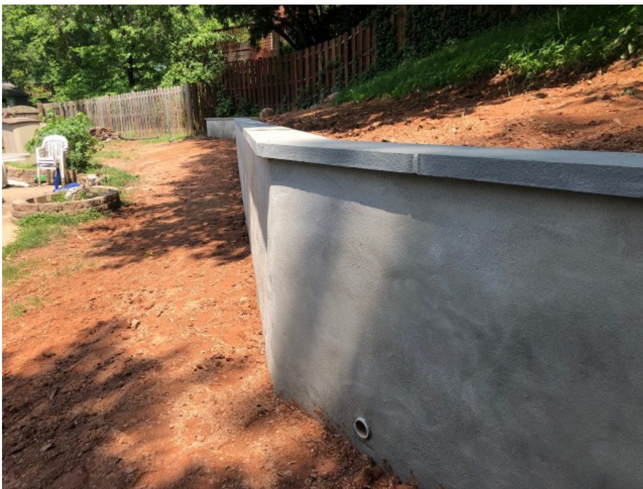
Block Wall with Parging
