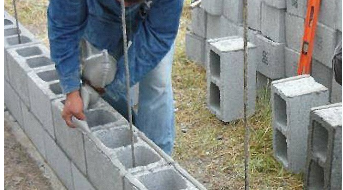
Block wall construction
