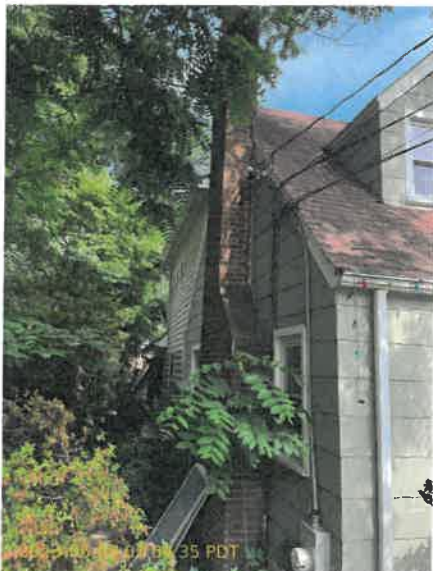
Utility Side Before Installation
