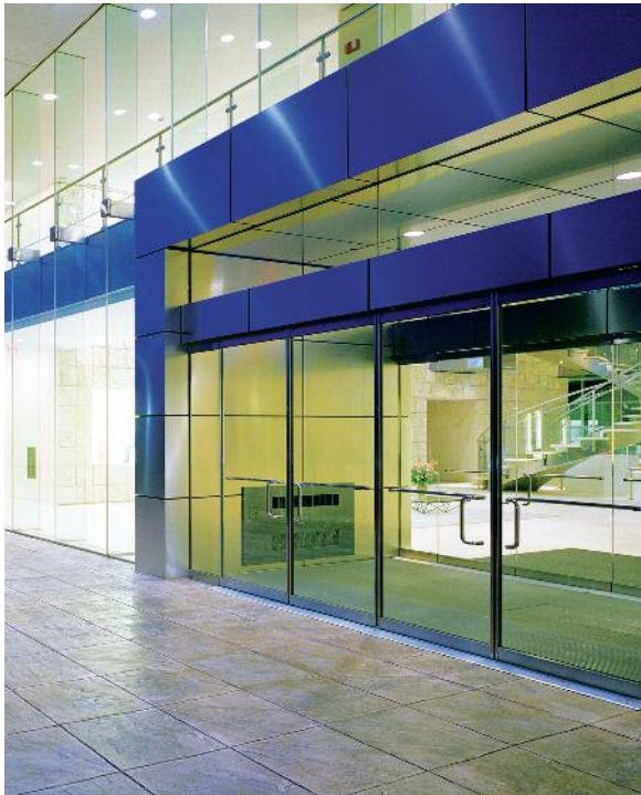
Jackson National Life, Lansing, MI Architect: Smith, Hinchman & Grylls Associates
