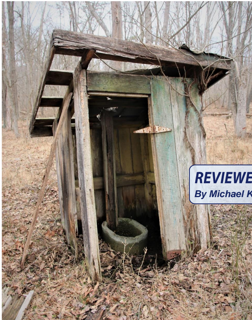
Front view (facing school) door and part of roof missing and deteriorated beyond repair
