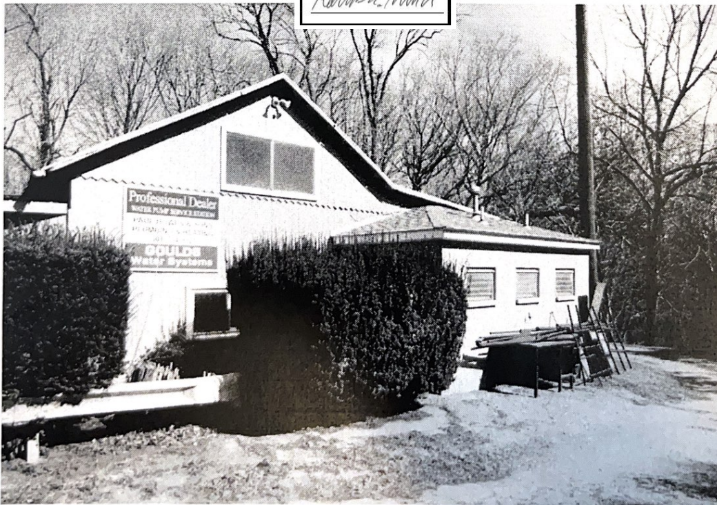
Figure 2 Existing south facade.
