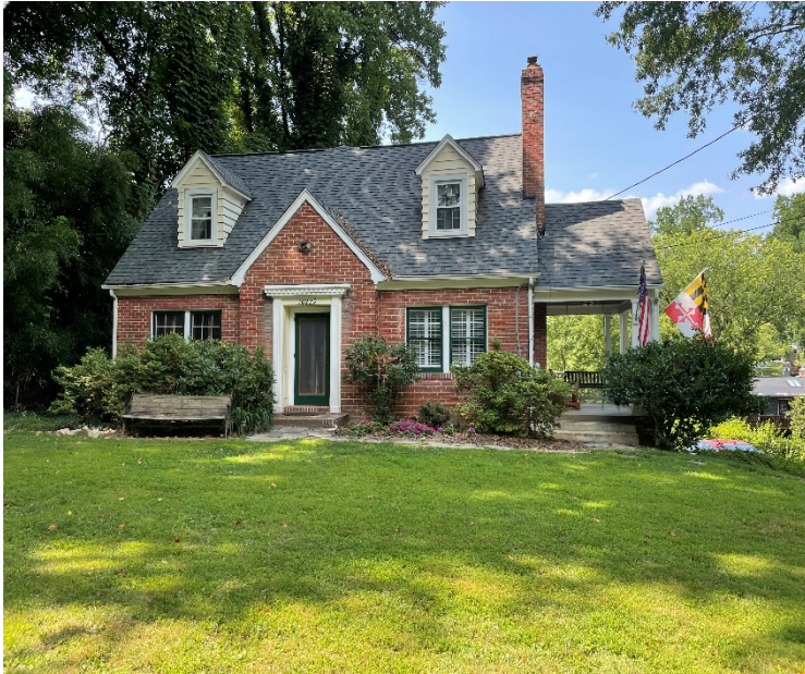
10229 Capitol View Avenue – single family dwelling
