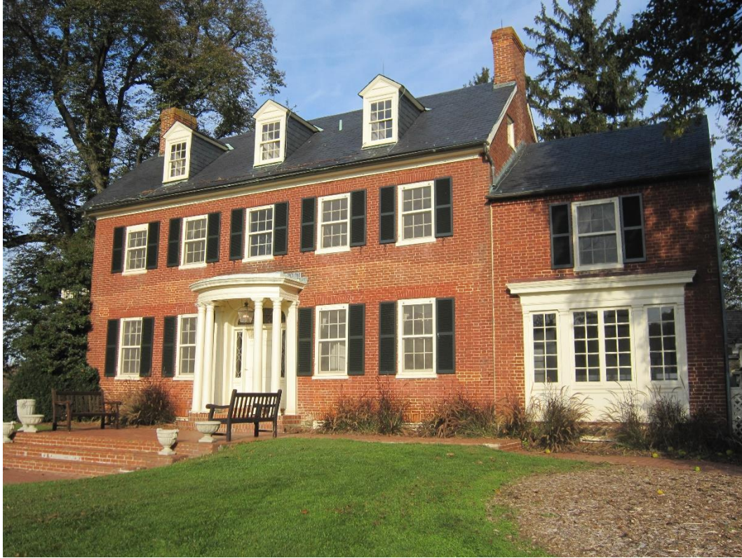
Woodlawn, front (south) elevation. Mudroom is not visible from this elevation.
