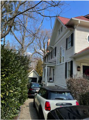
VIEW FROM WEST KIRKE ST. - LEFT SIDE
