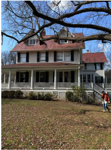
VIEW FROM SIDE YARD. - RIGHT SIDE
