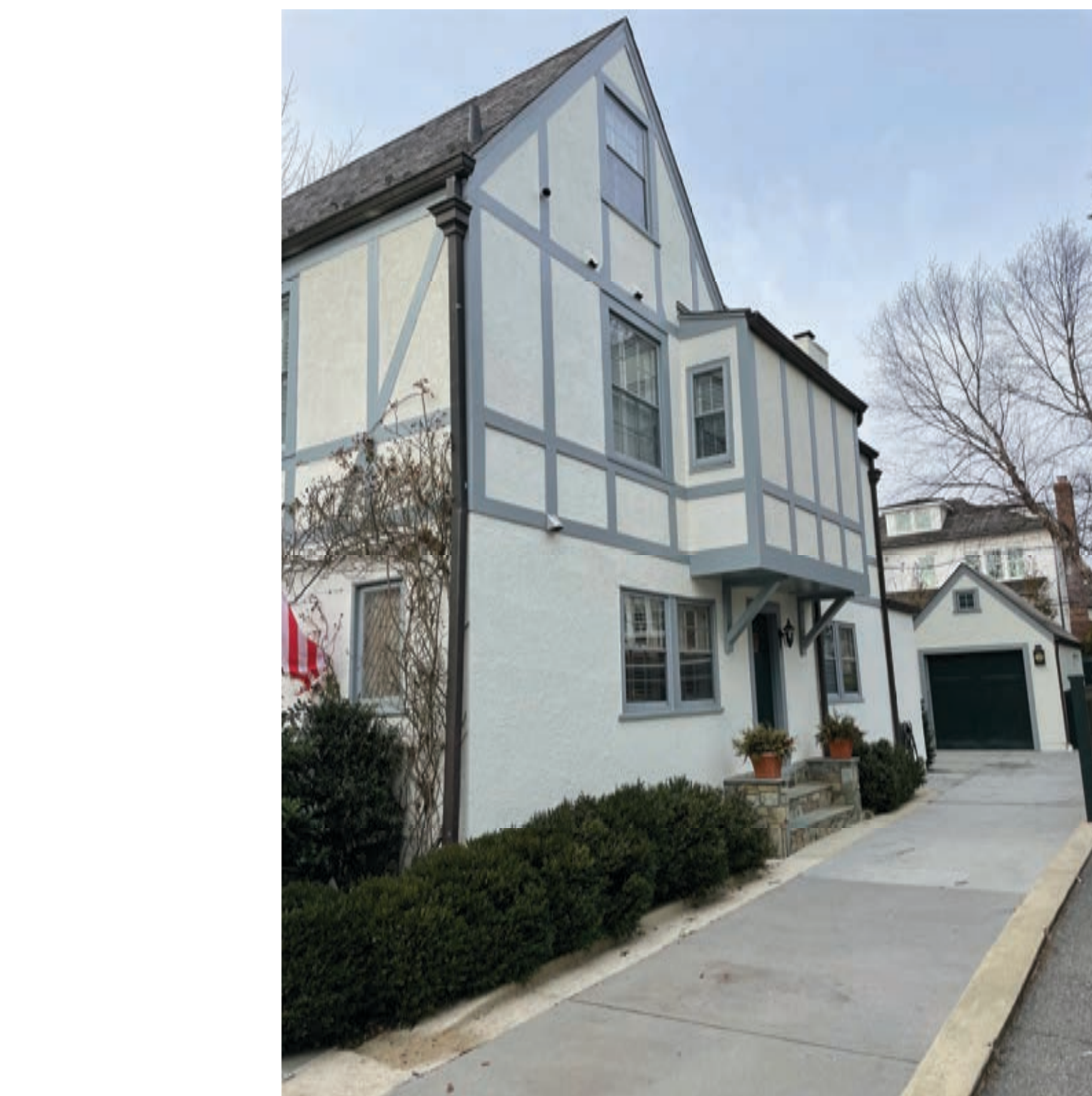
2. EXISTING EAST SIDE YARD
