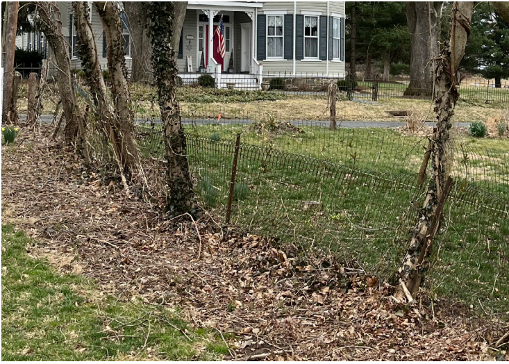
old wire fence
