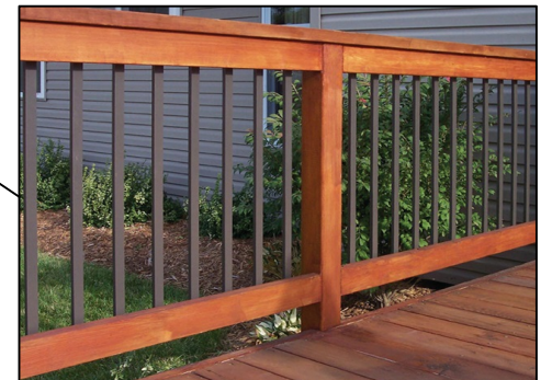
DECK RAILING OPTION- METAL BALUSTER OR ALL WOOD AND REPLACE 'IN KIND' IF METAL IS NOT PERMISSIBLE
