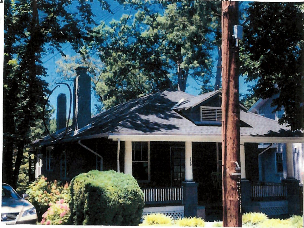
Views of front of 220 Park Ave small, second chimney is at the rear
