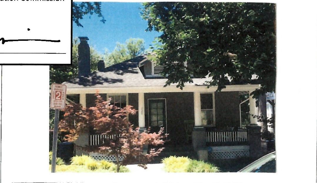
Detail: View from front of 220 Park Ave We'd like to remove the 2nd chimney in the rear of our home.
