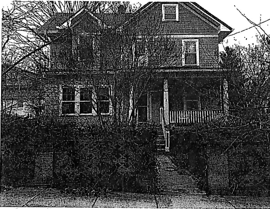
Detail: Front of house and CMU wall
