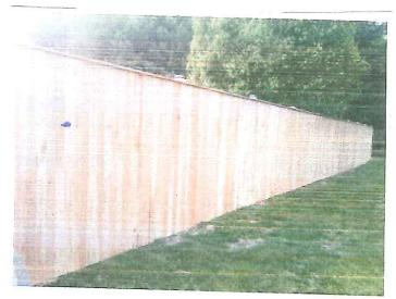
B-5' tall, pressure - treated pine, 4-board paddock fence (center back + right side to garage) with 2"x4" black viny (coated welded wire mesh; approx 156'
