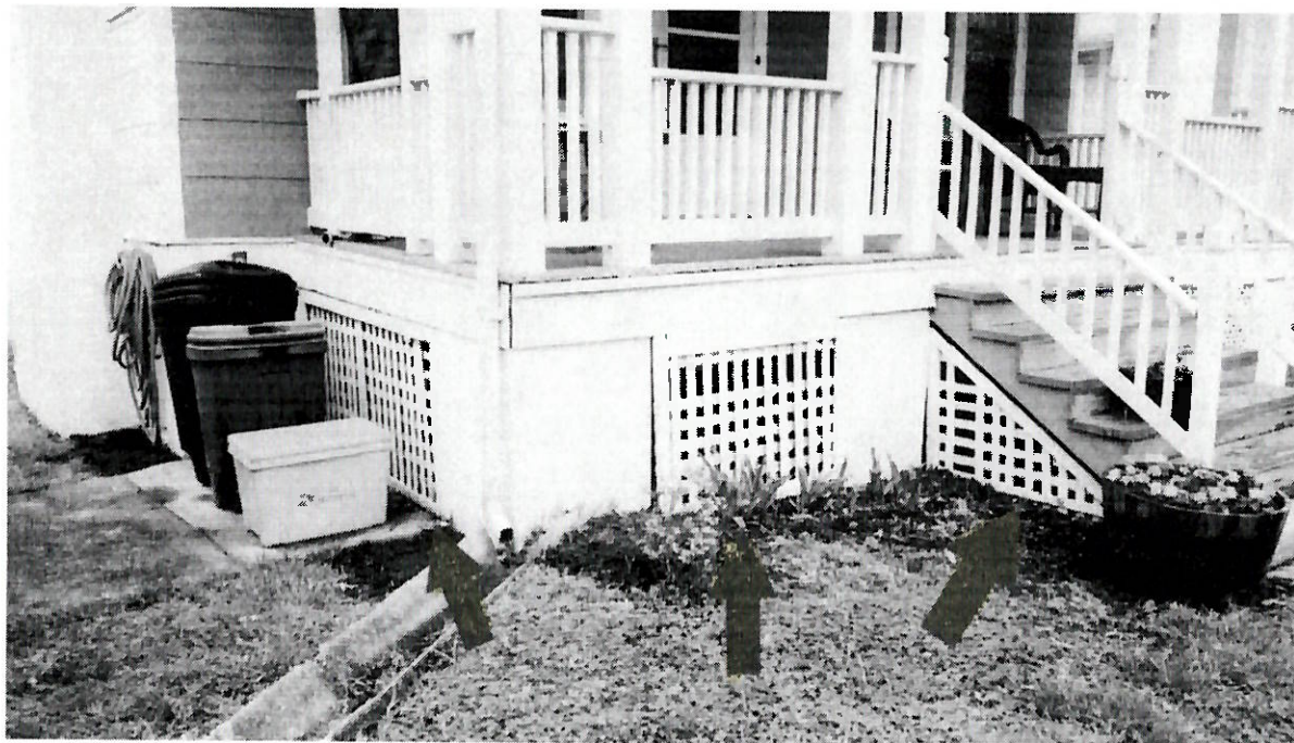
Detail: Figure 2. Original trellis / lattice on west side to be used as template and replaced. Note that there are vertical and horizontal bars missing due to deterioration rather than design.
