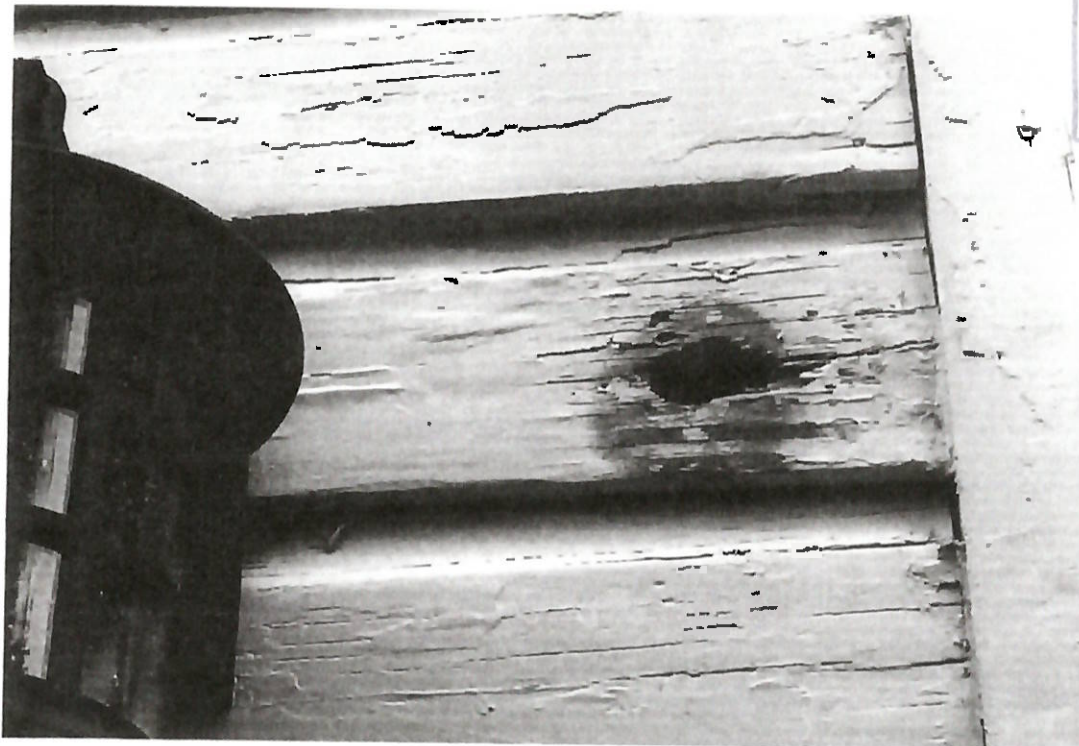
TYPICAL WOOD SIDING (TO BE RESTORED, REPAIRED, REPLACED) AND TRIM
