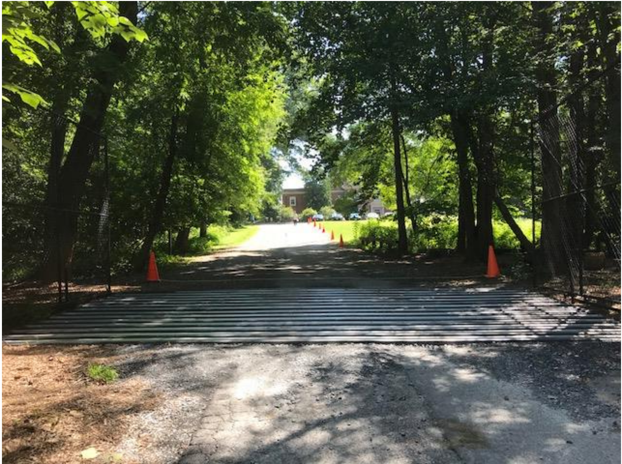
Existing cattle gates and fence at Brierly Road Exit
