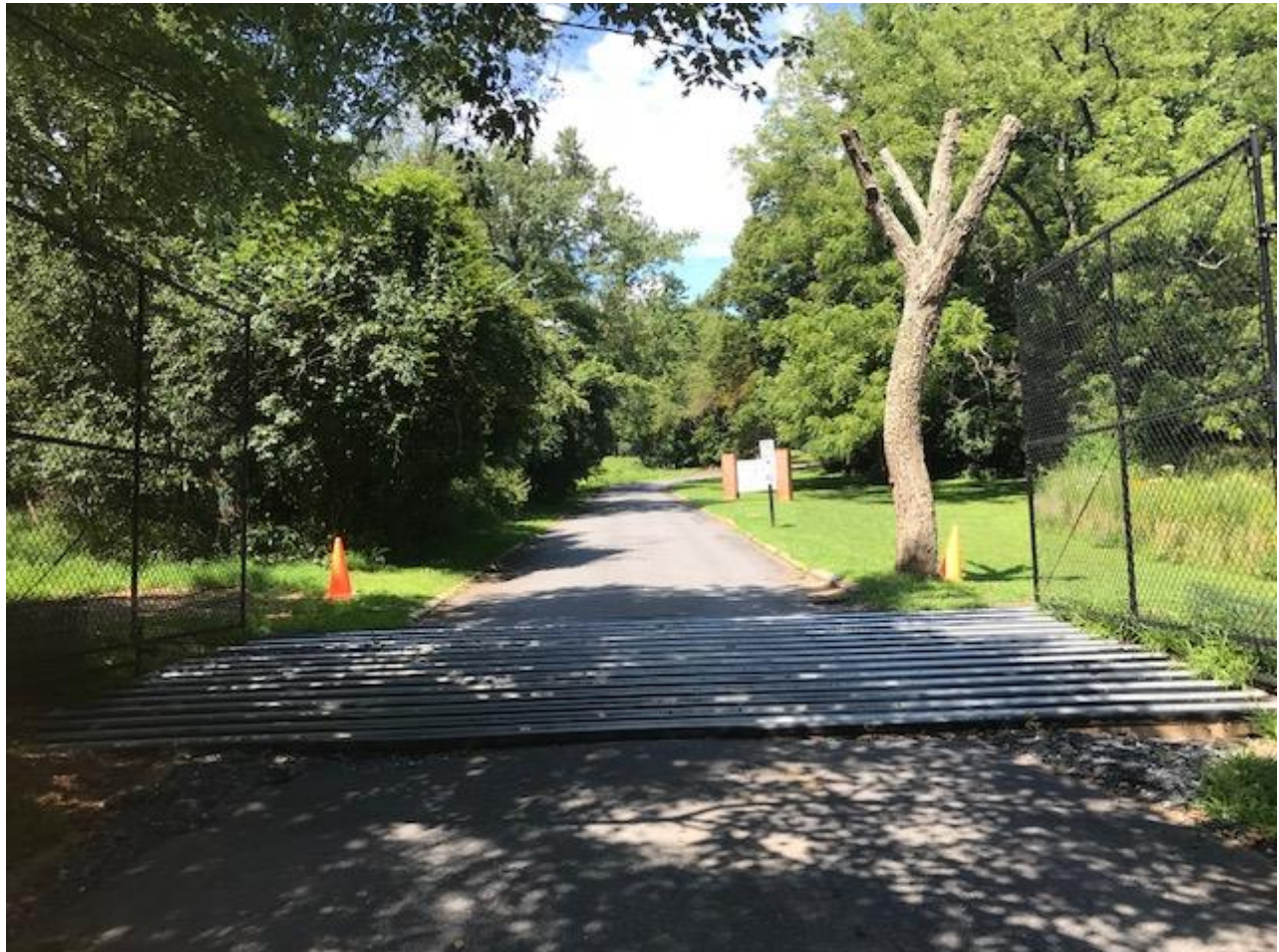
Existing cattle grates and fence at Jones Mill Road Entrance
