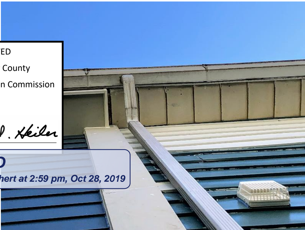
View of non-historic aluminum soffit and new wood soffit for addition
