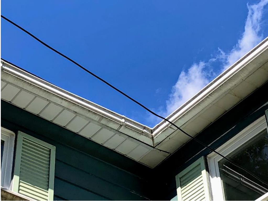
View of non-historic aluminum eave soffit
