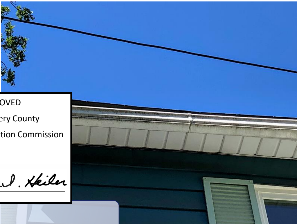
view of non-historic aluminum eave and rake soffits
