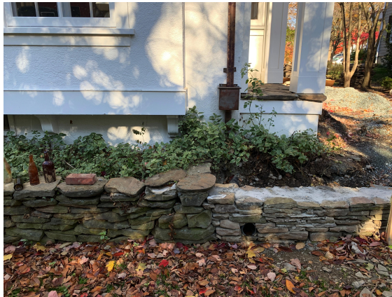
EXISTING WALL (LEFT); NEW WALL (RIGHT)
