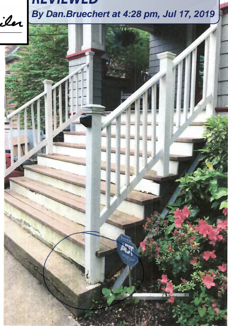
close-up to show rise of step is unnaturally high, creating a trip hazard
