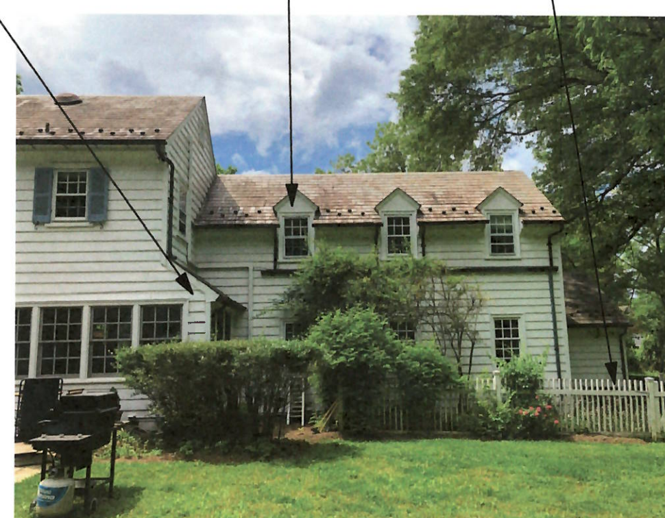
View of Rear (East) Facade
