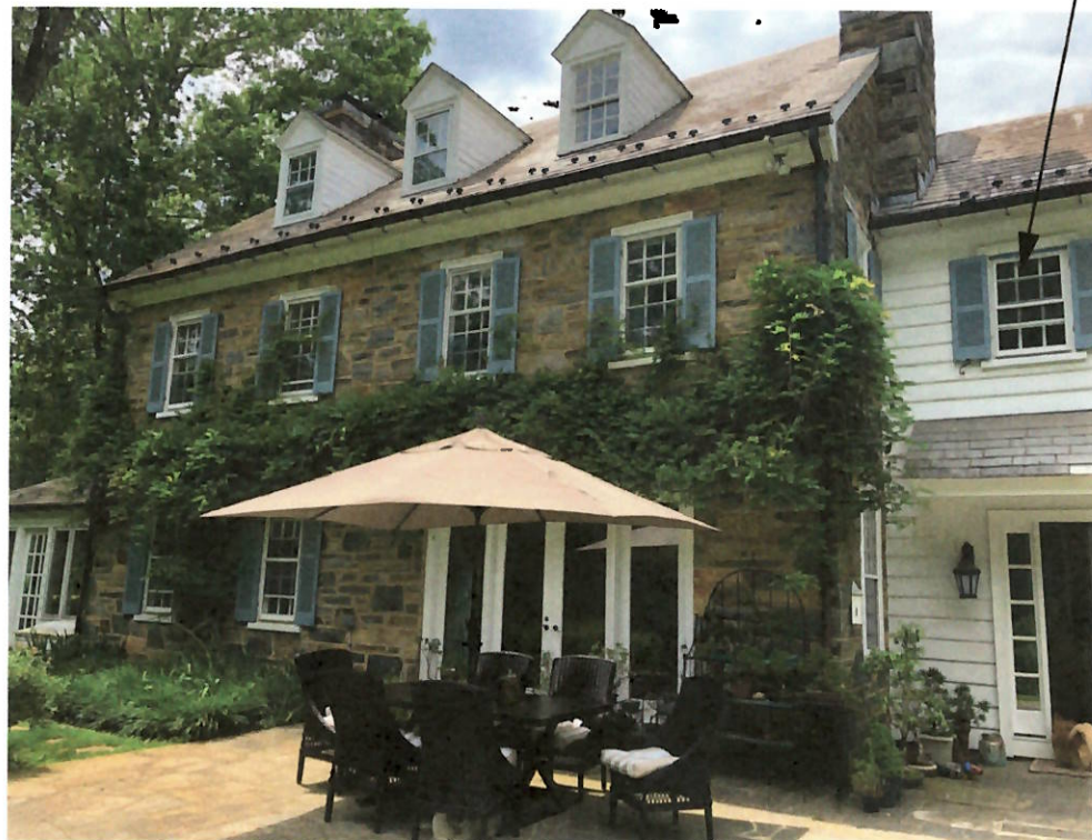
View of Rear (East) Facade
