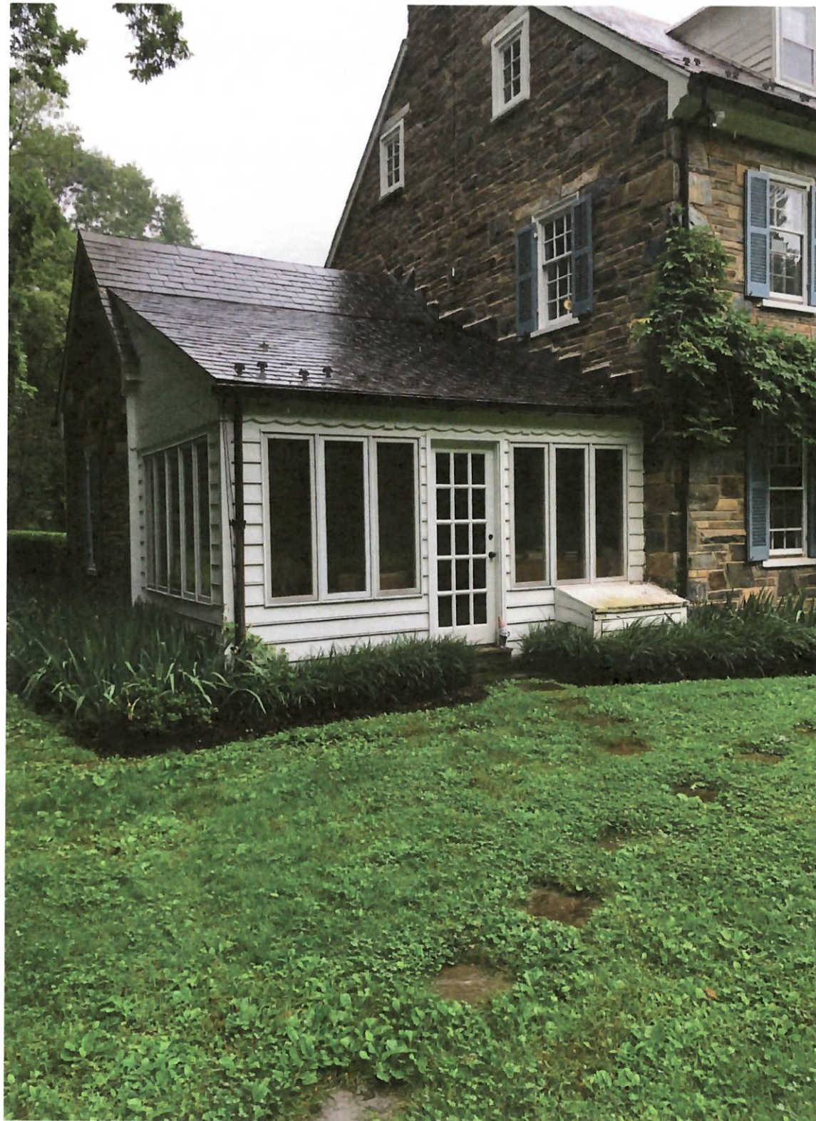
View of Ex. South Facade
