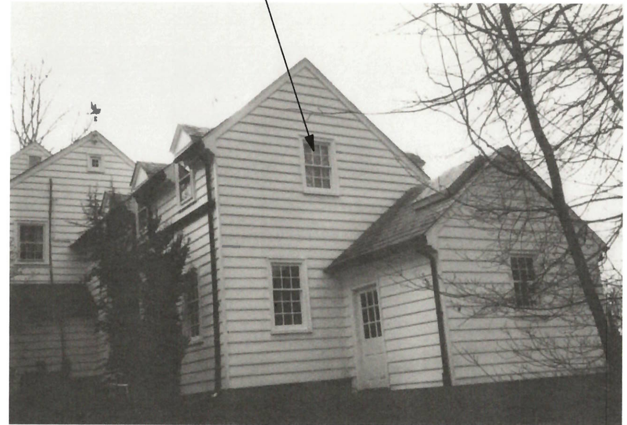
View of Ex. North Facade
