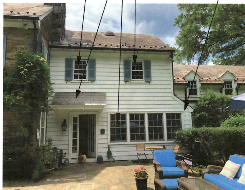
View of Rear (East) Facade
